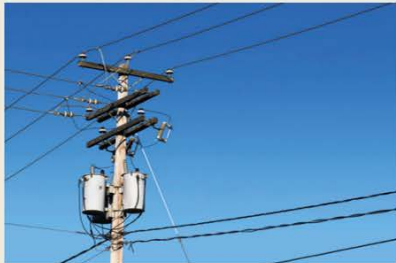
FIGURE 14.2.15 Electric power line poles carry the current and power to houses, hold transformers (grey boxes), and sometimes carry telephone cables.
